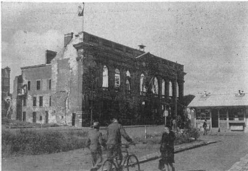
Only a shell remains of the city hall in Beauvais
