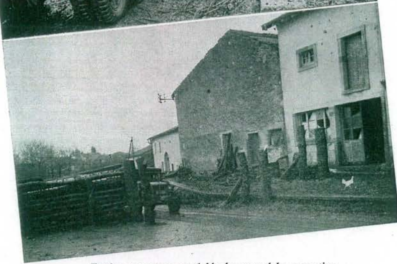
Engineers remove road blocks erected by retreating Germans near Montigny.
