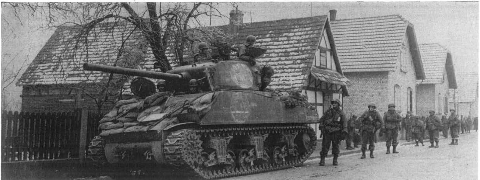
Advancing through Rohrwiler
